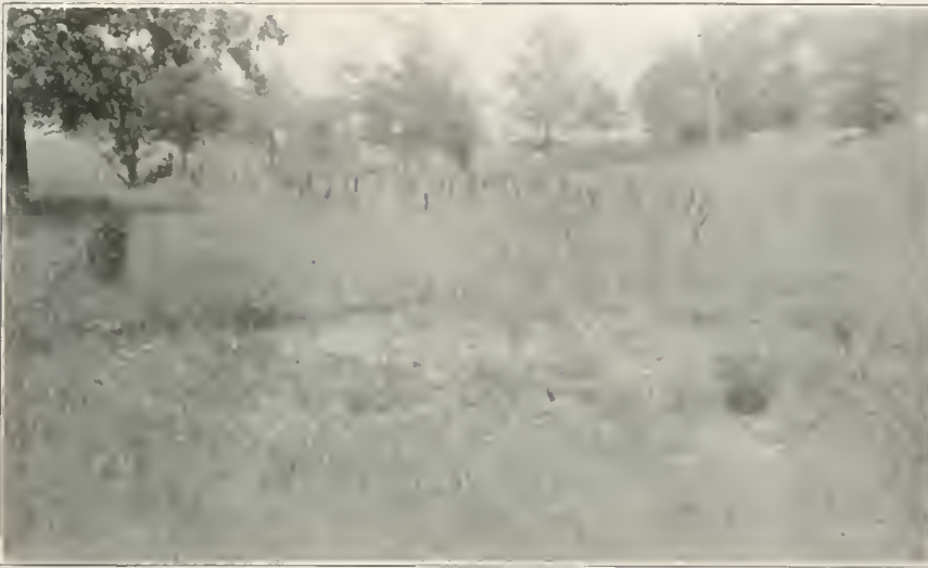
No. 8. Pot hole filled with brush and earth. The brush was used to prevent the earth being washed out during heavy rainfalls
